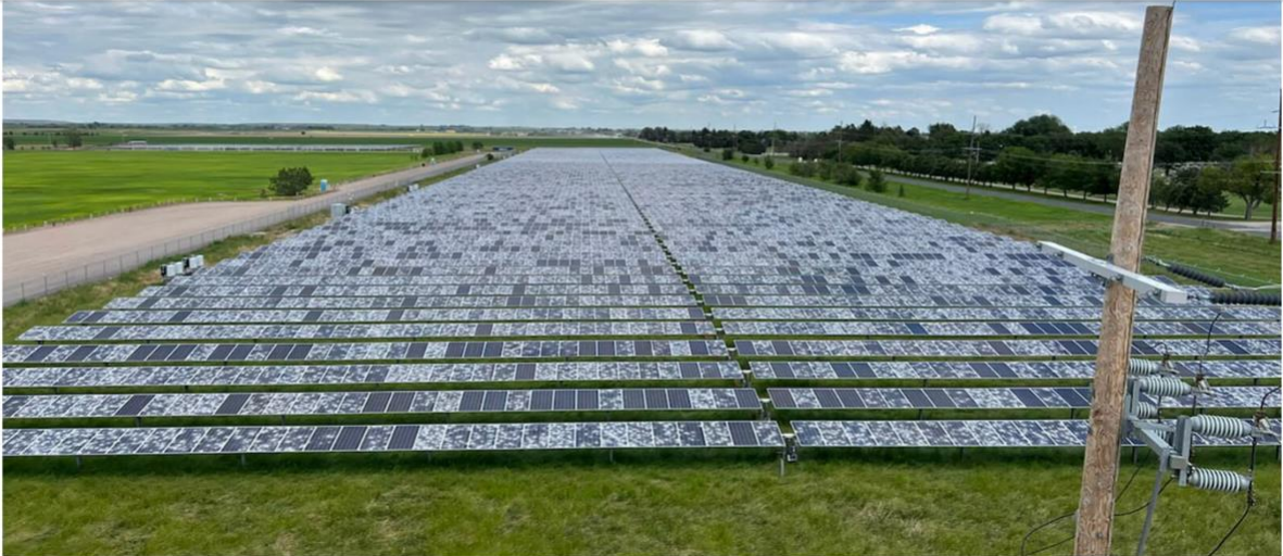
A solar farm near Scottsbluff, Nebraska, suffered major damage in June 2023 when a storm dropped baseball-sized hailstones at 100 to 150 mph on it. (Courtesy Photo)
