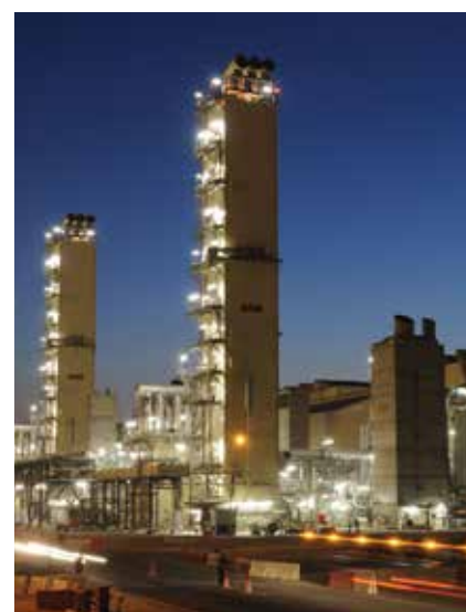
PEARL GTL, QATAR
