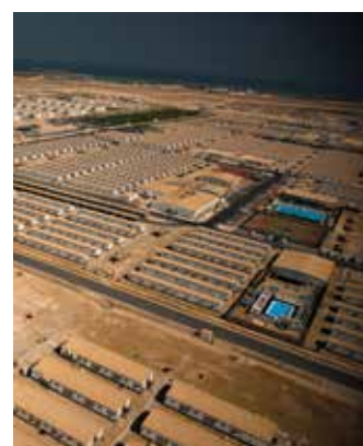
PEARL GTL, QATAR
